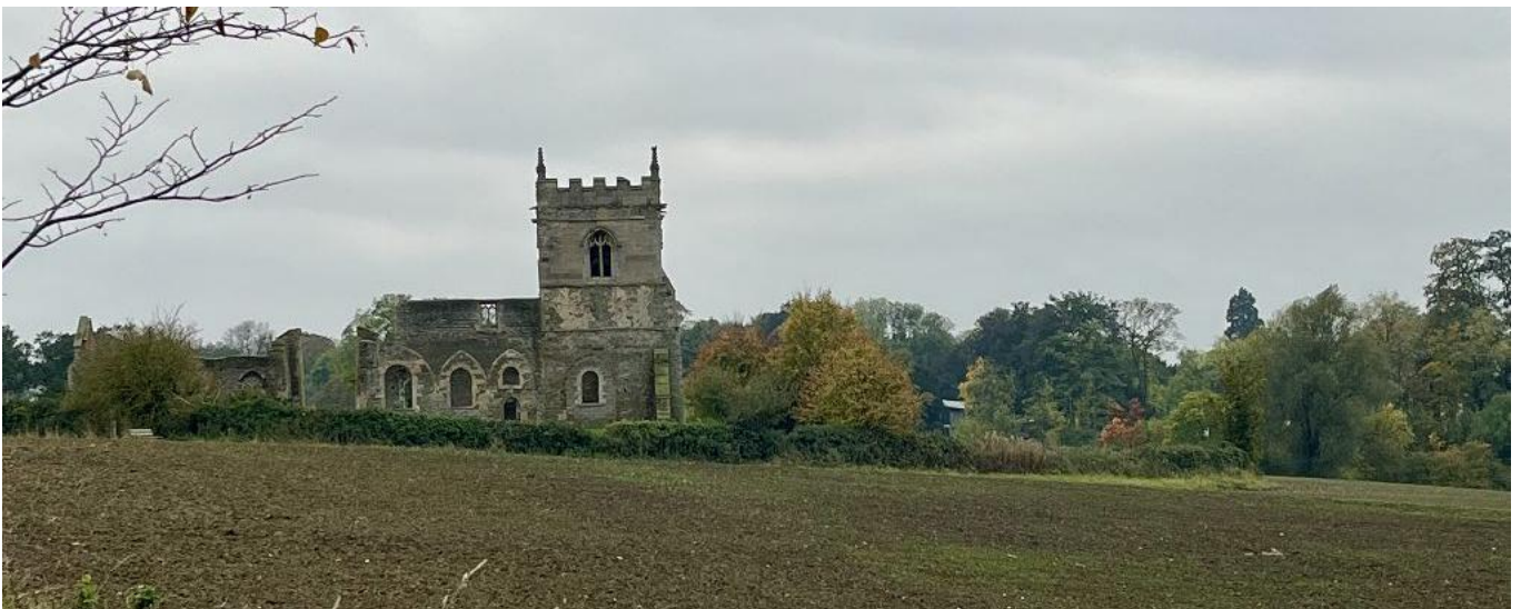
Figure 6 - View of the ruin of St Mary's Church from New Road
